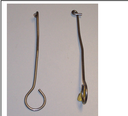
Pig-tail Wood frame brick tie - stainless
